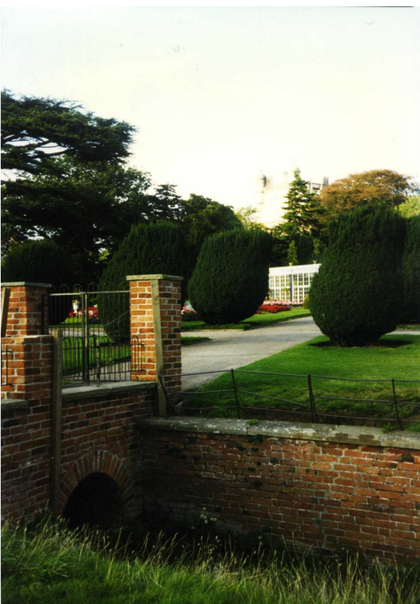
Figure 2: The ha-ha at Wollaton, Nottinghamshire; photographs taken by Richard Oliver in September 1997. The normal-sized bricks give an indication of scale
