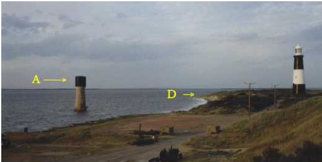
Figure 2. Looking from south of point 'B' on Figure 1 northwards, at equinocal High Water Springs on 24 September 1991. Observe tide-line at point 'D'. [© Richard Oliver: R.95/17A]
